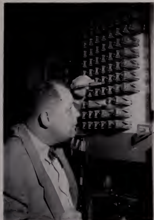
Jack McBrian, of Audio-Video Engineering, taking a close look at part of the complicated relay system for 6B, which was originally conceived by him.
