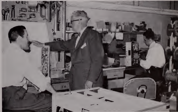
Frank Connolly, audio-video construction man (left) and Dave Moloney, technical construction superintendent, examining drawings associated with the TV Master Control installation. On the extreme right is Sal Salantro, audio-video construction man, building a monitor for kinescope recording.
