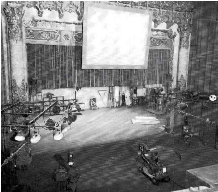
FIG. 1. View of the El Capitan stage and operating areas. An RCA PT-100A Theatre TV Projector is used to show the picture being transmitted on the large screen above the stage. Note the camera "pit" at the lower right.
