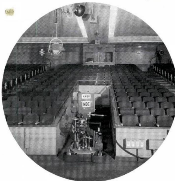
FIG. 1. Operating space of Studio D stage area includes this recess into audience seating area which allows movement of cameras for stage or audience shots.
