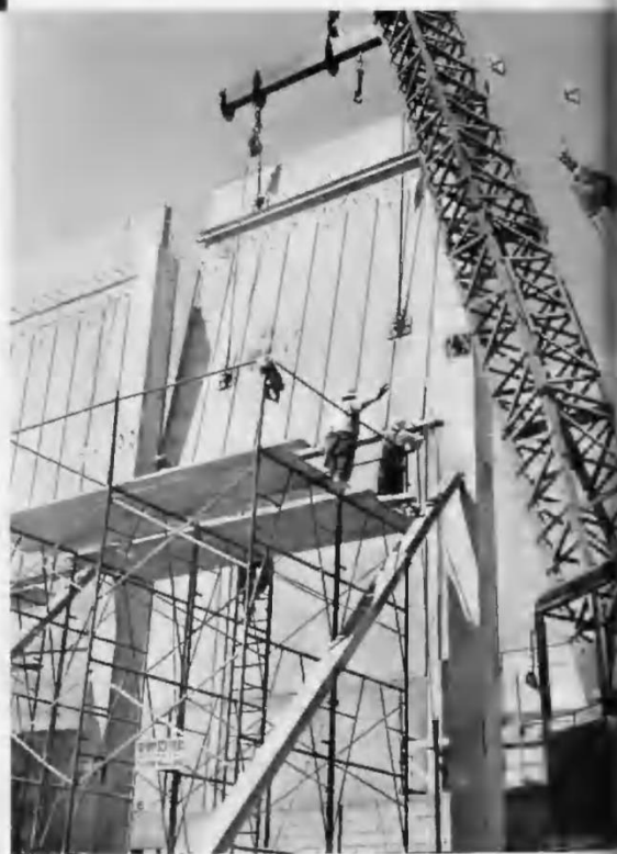
A huge crane swings a 16-ton concrete panel into place as part of the studio's outer wall.
